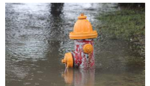
A fire hydrant on S. Hughes Street became a little soggy.
