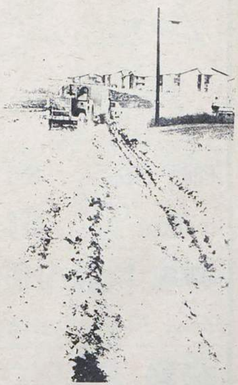
CITY PROJECTS--New six-inch water main approved by city council for the south part of Howe is in the process of installation (upper photo). The new larger main was approved to alleviate low water pressure in that area of the city. In lower photo, what appears to be a snow storm is actually lime being applied to West Haring Street in Western Hills after a portion of the street was plowed up in preparation for refinishing. Project caused closing of the street most of last Saturday.
