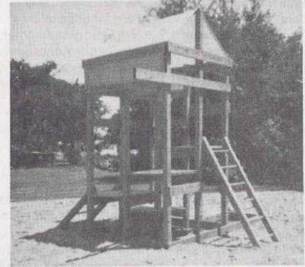
MEMORIAL PARK - Shown is park of the playground equipment being installed at the new park. Special thanks to Brent Lankford and the Howe Ag class who helped assemble it.
