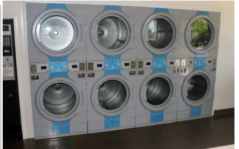
Eight of 14 new dryers have been installed at Howe Clean! the newest laundromat in Howe. It is scheduled to open later this week.
