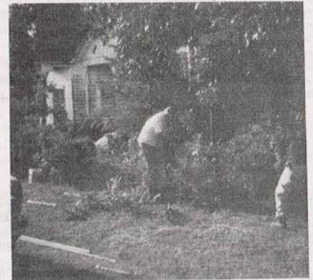
TAKING DOWN THE FENCE - Workers for the Howe Chamber of Commerce took down the fence at the house on the corner of Kosse and College. The fence will be used at the city's Memorial Park on Denney St.
