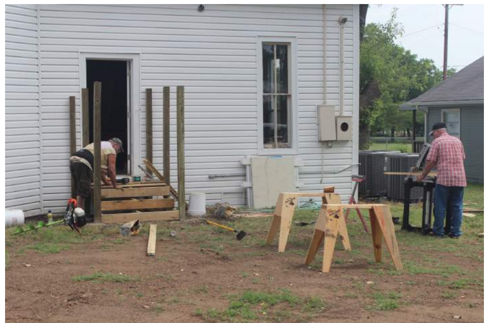
Mike Barlow (left) and Boyd Dunn (right) build a back porch at Summit Gardens.
