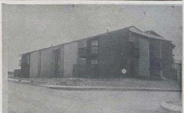
Eight of 100 apartment units are contained in the building above, with 32 units, or four buildings, completed and ready for occupancy. Complex also contains a recreation building and playground.
