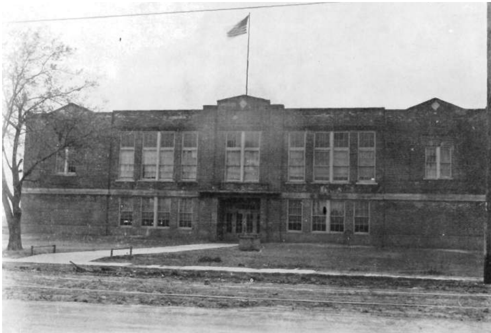
Marshall-Bean College located at the present location of the 1938 WPA Howe school (now administration office) on Denny Street.
