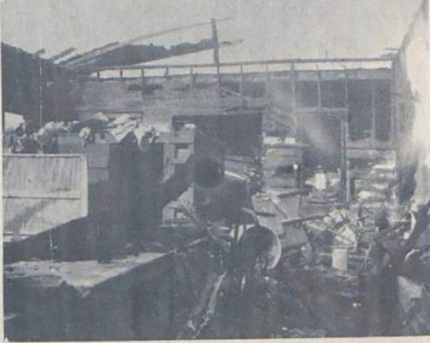
Gutted interior of Davis Honey Co. building following fire
