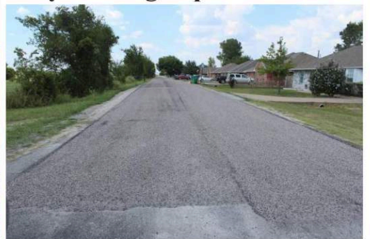
Farmington Road completely resurfaced
