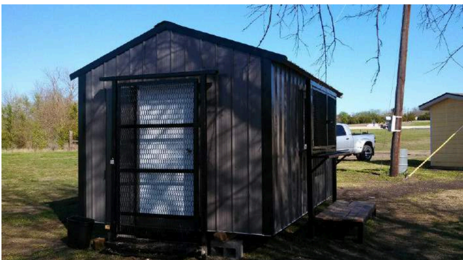
The "prison gate" on the concession stand at the North Field prior to vandalism.
