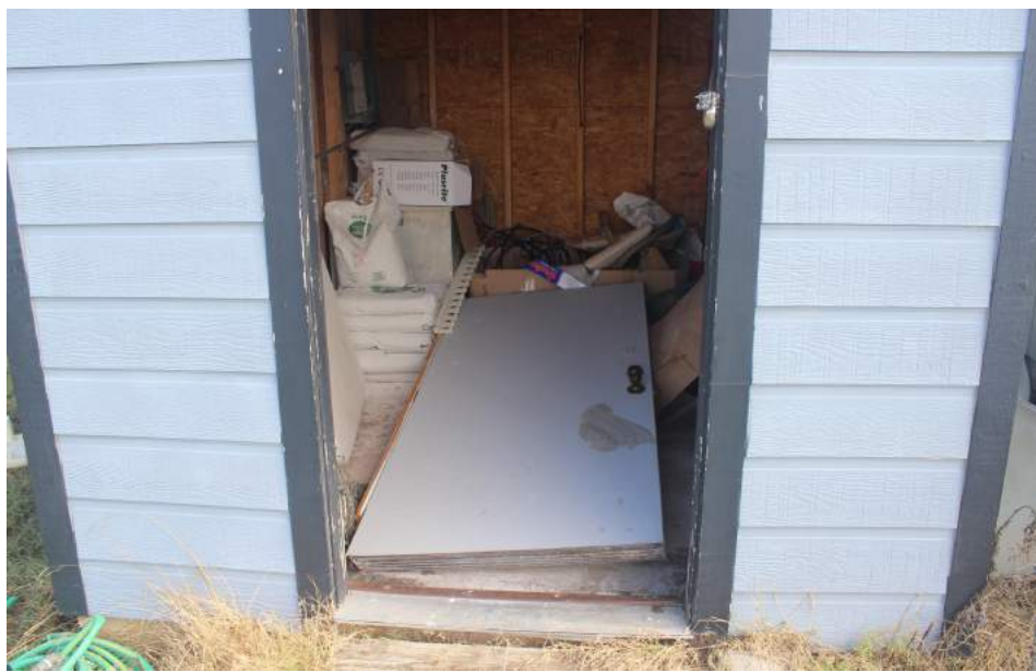
The door kicked in at the North Field storage building.
