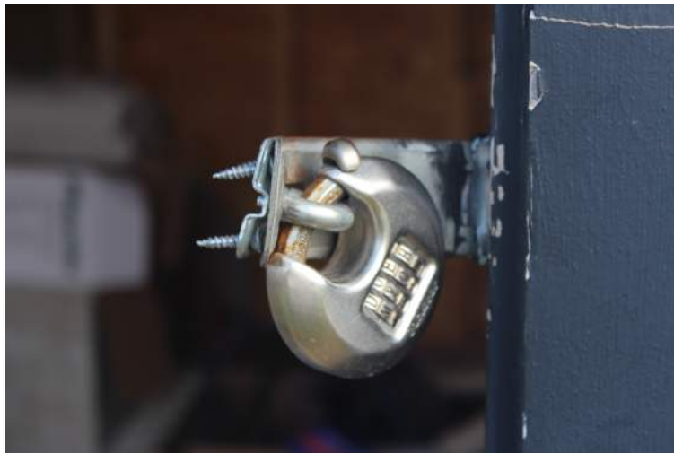
A latch that was destroyed at North Field in Bi-Centennial Park.
