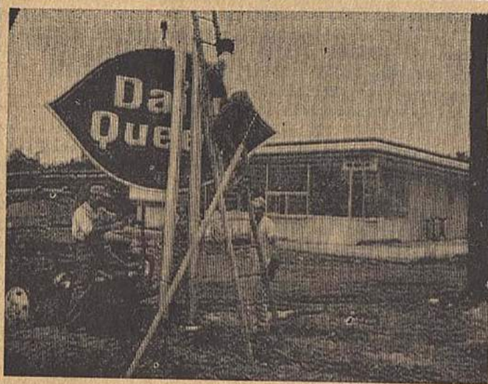
GOING UP — This was the scene earlier this week at the location of the new Dairy Queen Store in Howe. Workmen hoisted the huge sign into place in preparation for the Grand Opening Saturday. Arnold Sasser, operator, said the new store would be open Friday afternoon in order to test all the new equipment.
