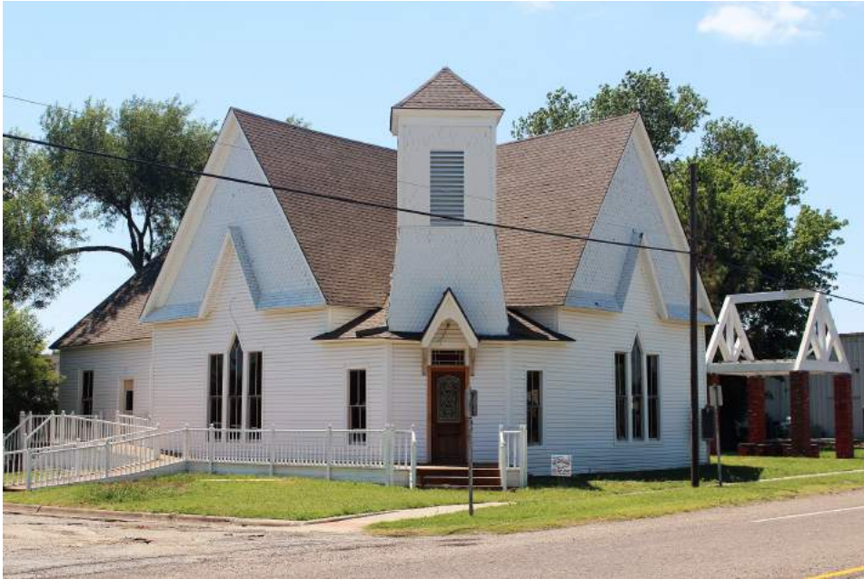
The 124-year-old former First Christian Church, now Summit Gardens, received a new roof last week.
