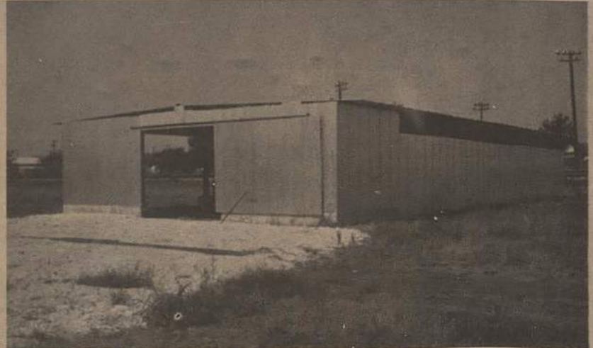
New Vocational Ag Building Under Construction
