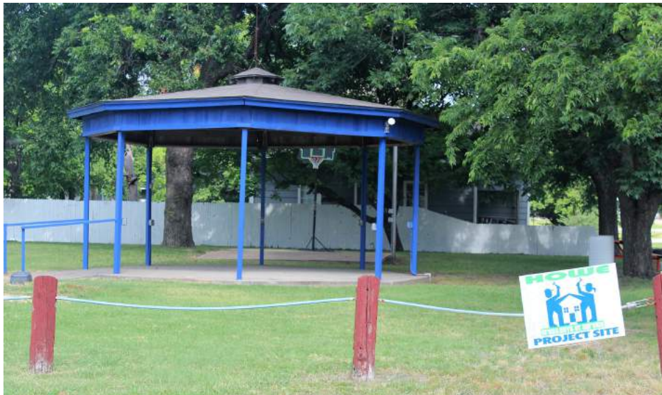
The finished product at Memorial Park. The gazebo was painted blue from red and the fence to white. A basketball goal was also installed.
