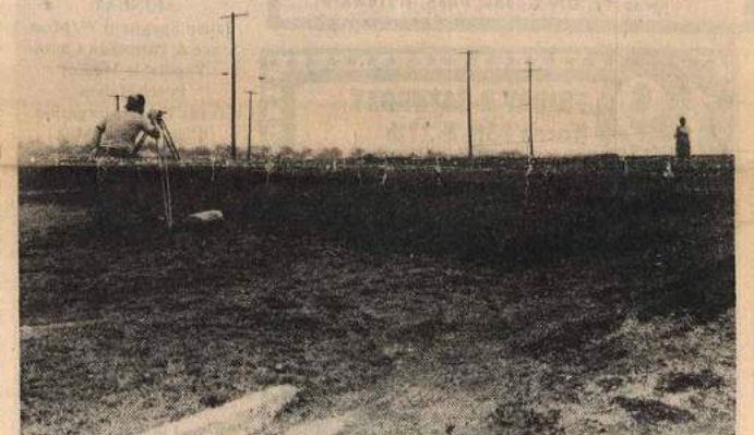
A TERRACE was built east of Western Hills Drive to help alleviate a drainage problem that has been causing large amounts of mud to accumulate on the street during rainy weather.
