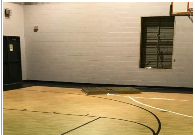
Destruction of vents in auxiliary gym.
