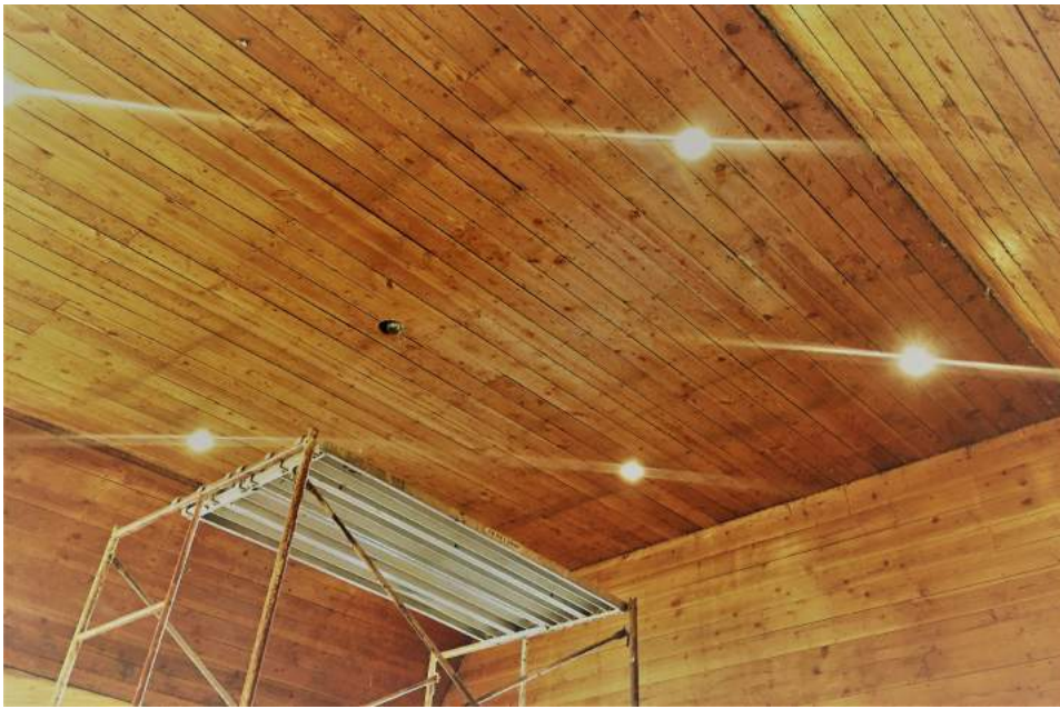
Can lights have been placed throughout the interior of the old First Christian Church.
