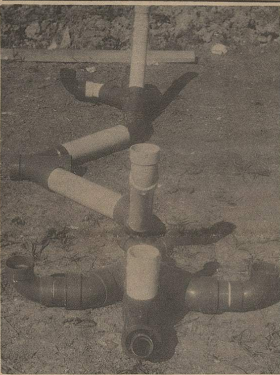
This is what it appears to be, if you're familiar with this type thing. It's a bunch of assembled plumbing for one of the apartment buildings under construction in Western Hills. Fourteen buildings to house 100 units is currently under construction with completion set about September, 1972
