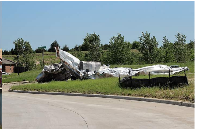
The roof of the Tapia home relocated to Summit Hill.
