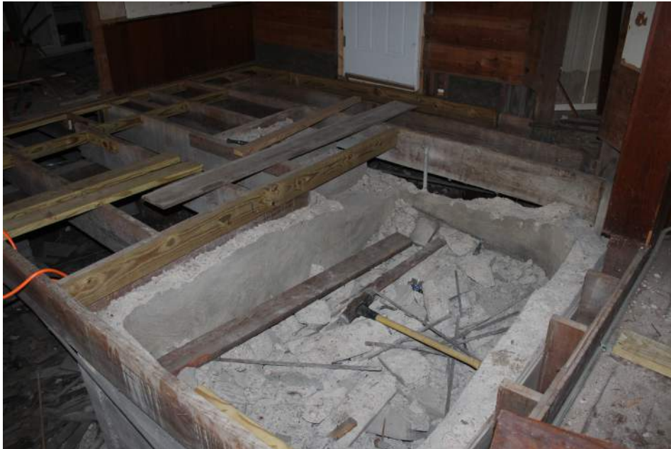
Remains of the baptistry that had to be cut out
